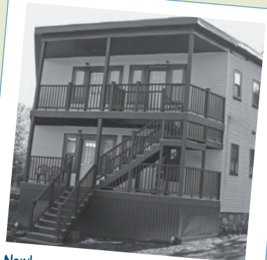
Newly renovated porch on the back of HCA's Peirce property
